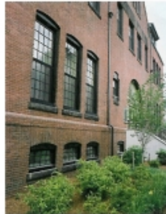
Photos courtesy of Sea-Dar Construction
